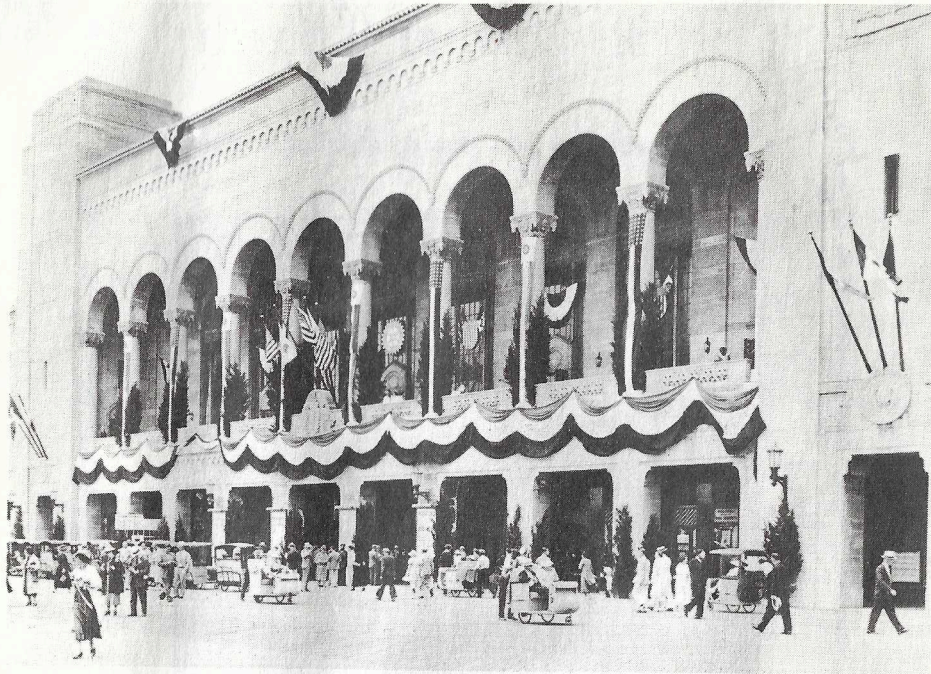
Boardwalk Front of the Atlantic City Convention Hall
